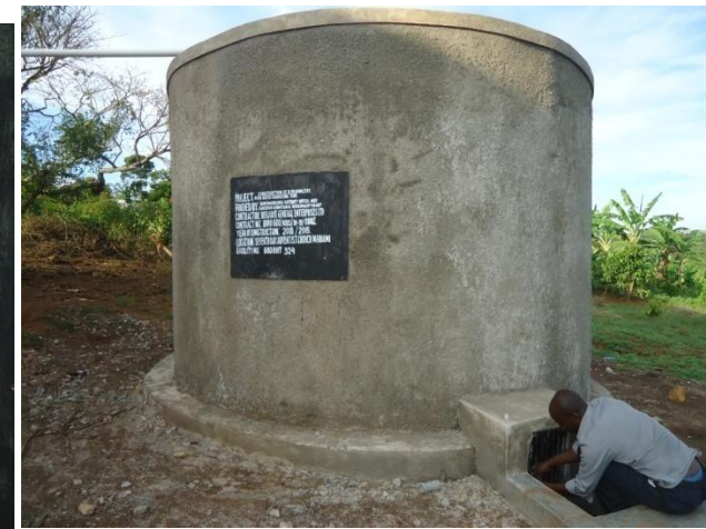
Below: 30,000 Ltrs Rainwater harvesting tank at Seventh day Adventist Church Makomi P/S Bigasa.
