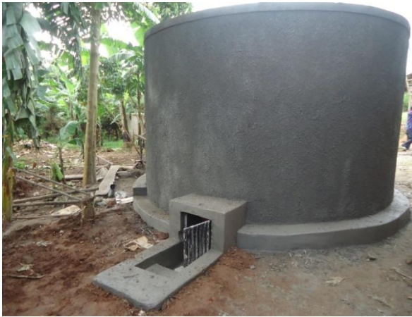
Above: Commissioning a 30,000 Ltrs Rainwater harvesting tank at St. Bernard Kateera P/S, Kibinge
